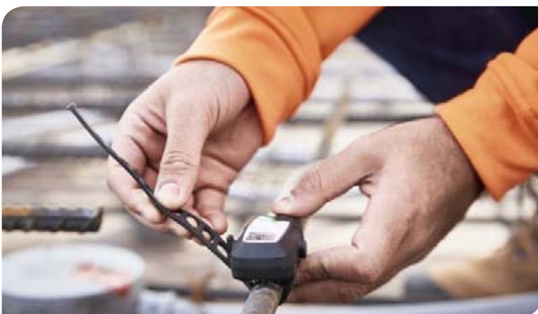
Below: SmartRock™ active sensor installation on rebar.
